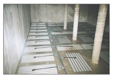
After the waste receiving has been expanded, a third underground aeration tank was built in 2014, wherein 49 MESSNER® Aeration Panels were installed. This is equivalent to 55% tank bottom coverage (refer to the picture on the left). At the same time the process engineering was optimized by implementation of a new interactive control system completely integrated in the existing PLC. Today MESSNER® ICS is controlling each aeration tank individually. This
