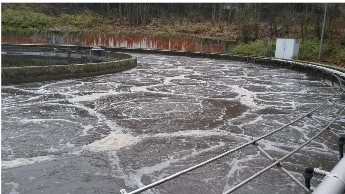
RMU Plug Flow Technology without agitators - wastewater treatment plant Bad Münster am Stein-Eberburg
